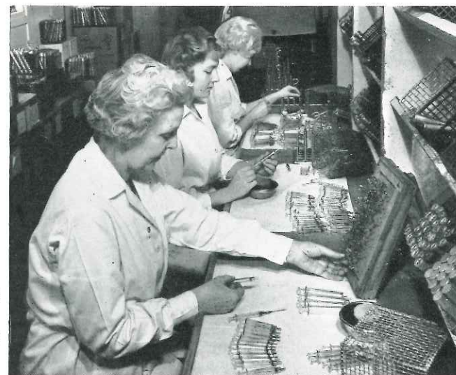
THE SYRINGES BEING LUBRICATED, ASSEMBLED AND MOUNTED WITH NEEDLES BEFORE BEING PLACED IN THE ALUMINIUM CONTAINERS.
